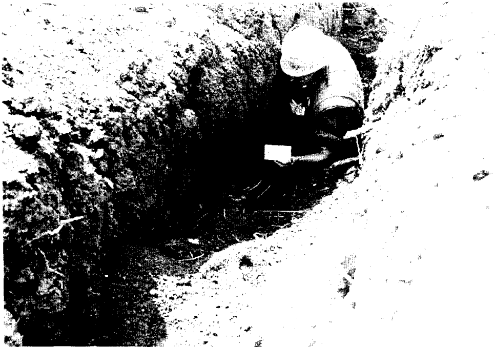
F-11 Protective Hole in Trenchline
