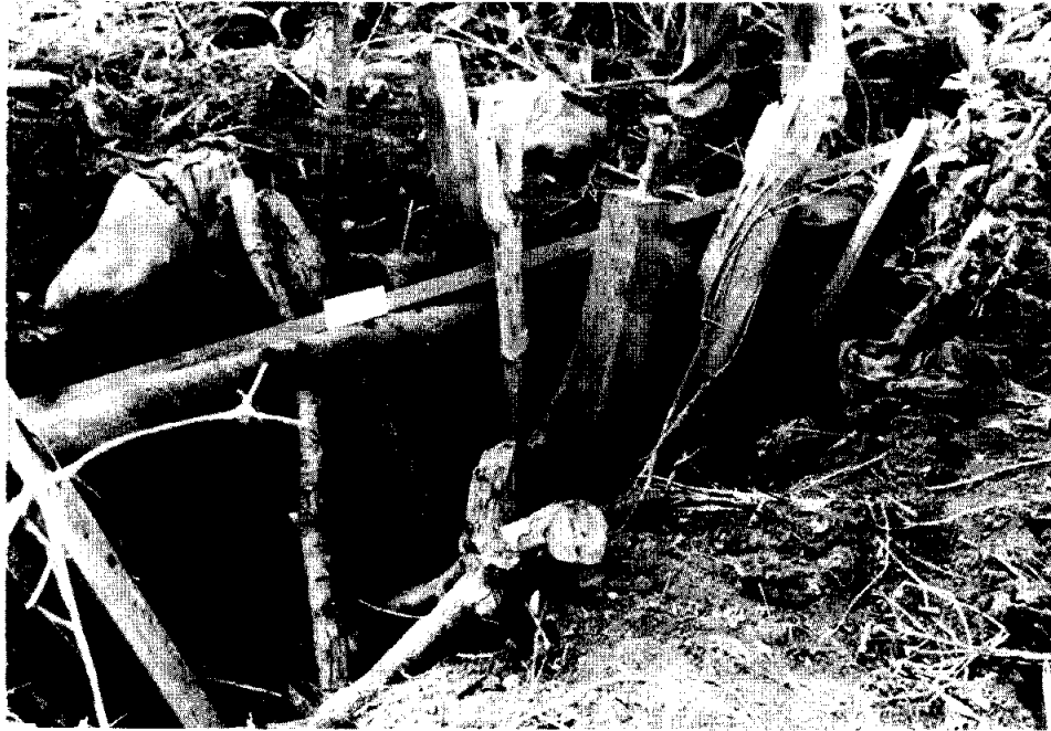
E-11 Bunker Materials
